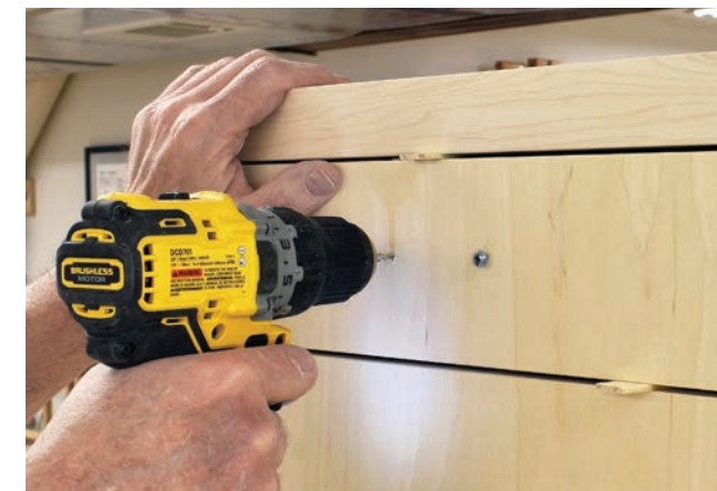
Use 1/8" shims to center the drawer face, then drill through the handle holes and into the drawer box. Bolts for the drawer pull hold the front in place until it's permanently attached with more screws from inside.
